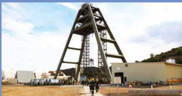
The A-frame over Shaft 10 at the Resolution Copper project outside Phoenix, Arizona, US.
